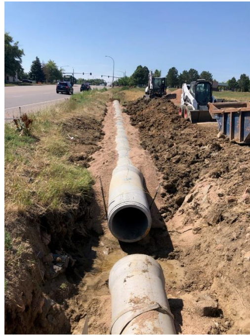
During: Installation of Pipe
