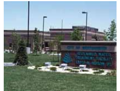
Big Dry Creek Reclaimed Plant.
