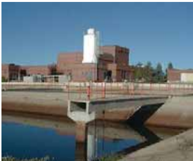
Above, an original rendering of the Big Dry Creek Waste Water Treatment Facility. Below, Semper Water Treatment Facility.
