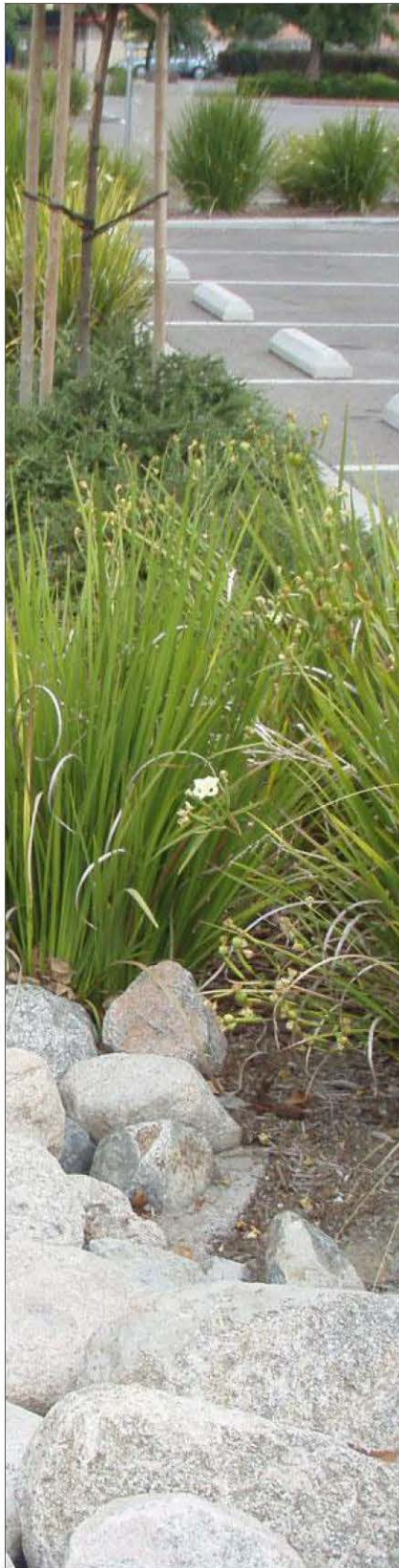
Parking Lot Bioswale
