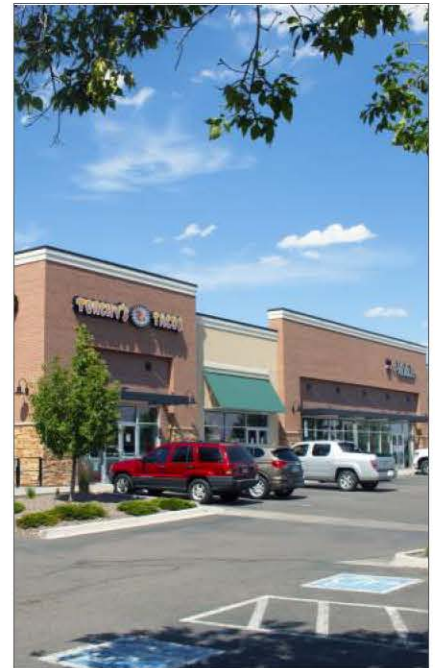
Towne Center at Brookhill
