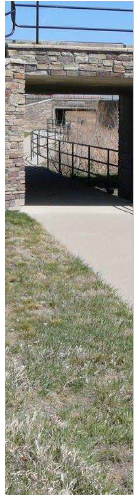
Huron Street Bridge and 142nd Avenue Circle Bridge over McKay Creek
