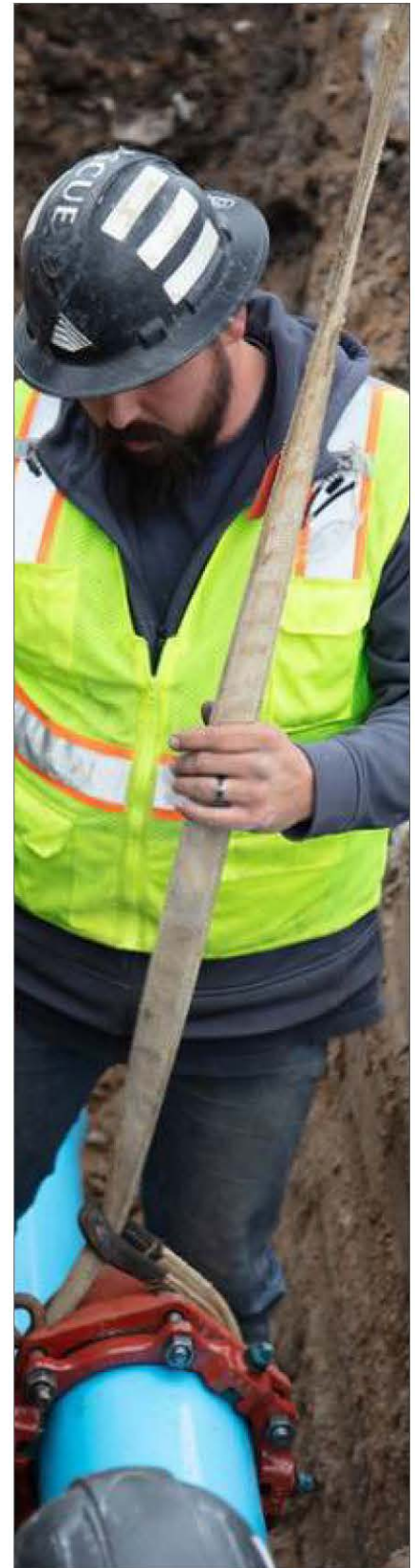
Water Main Replacement
