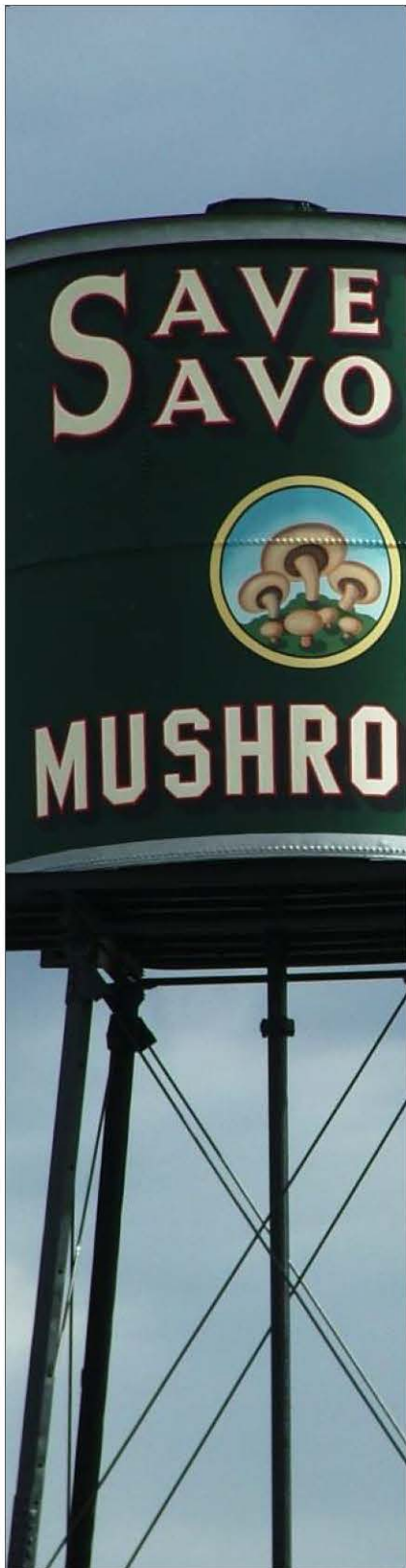
Restored Savery Savory Mushroom Water Tank
