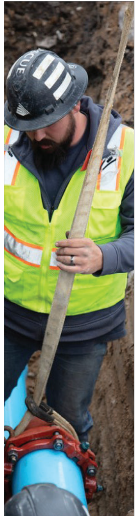
Water Main Replacement
