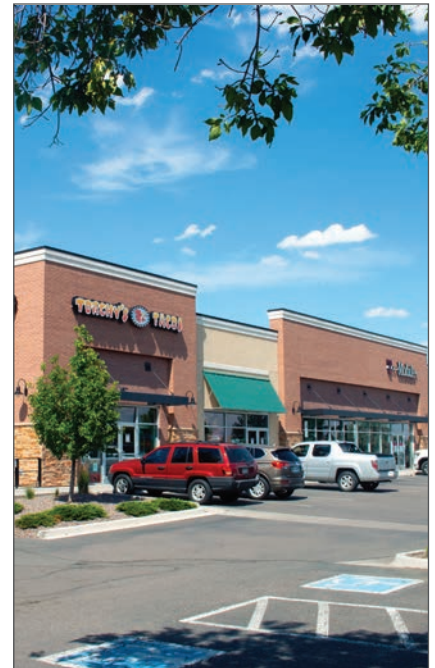
Towne Center at Brookhill
