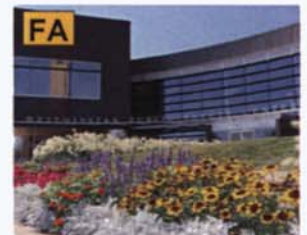
Fire Administration: 9110 Yates St. ■ -4500
